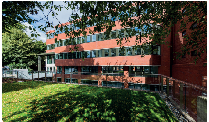
Two Haddington Buildings, Dublin (VSREE)
